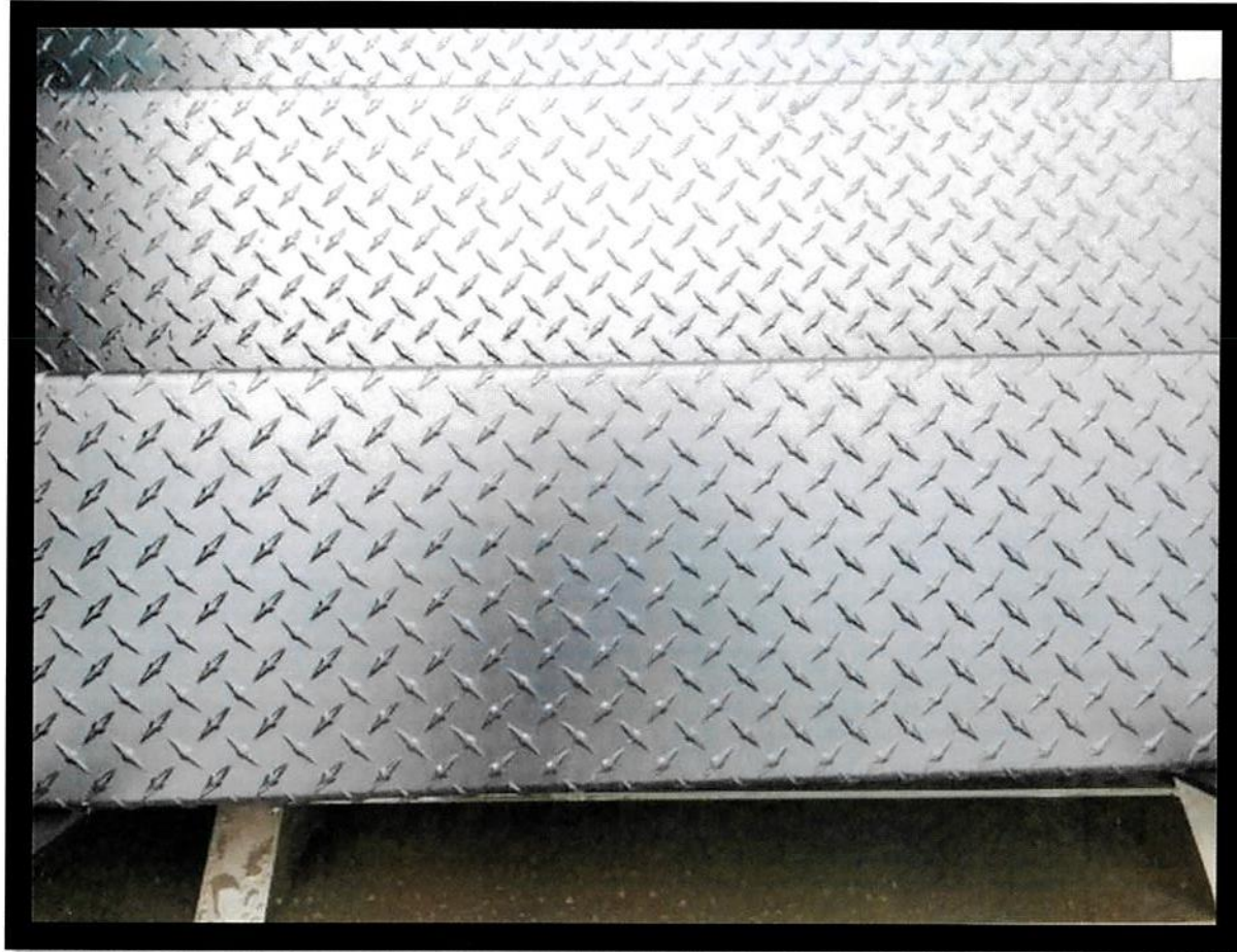
Checker Plate Stairs
